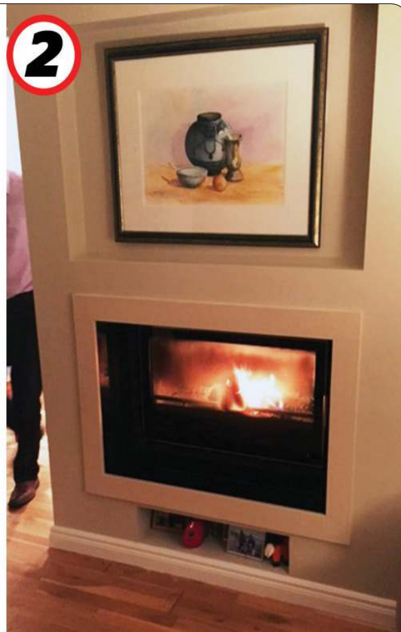
2 - COMPLETED INSTALL USING METAL STUD FRAME & HEAT RESISTANT PLASTERBOARD
