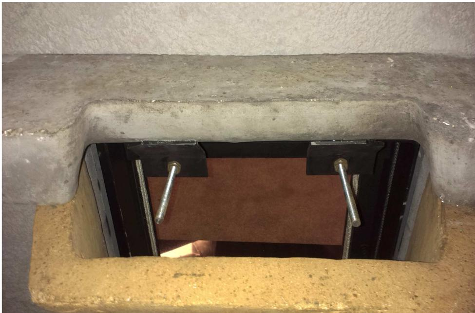
Fit the baffle to the top side of the door frame using the nuts, bolts and washers provided.
