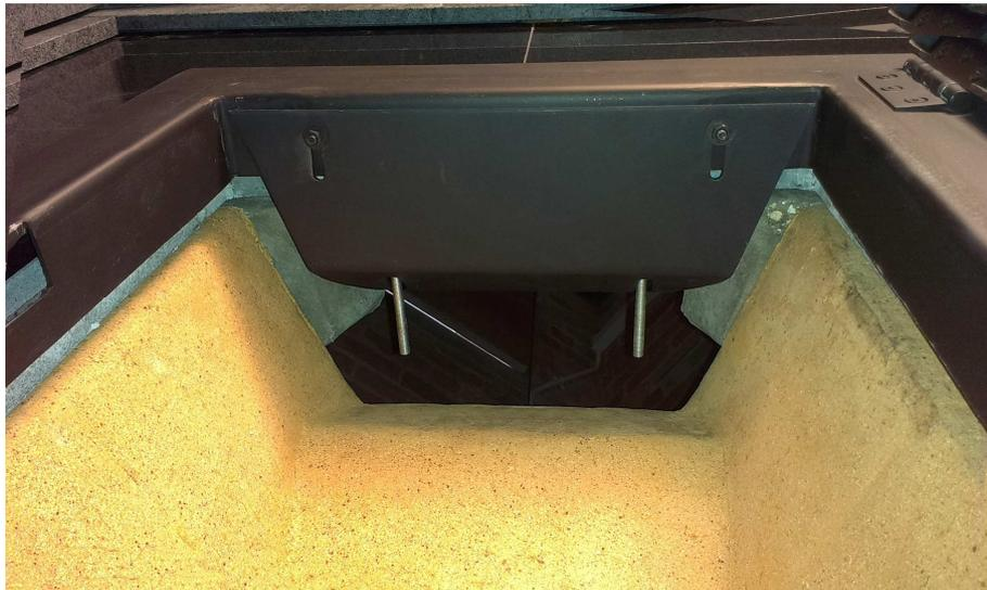
Fix the base of the door to the fireplace hearth using the 2 screw holes in the bottom of the frame. After fixing the base of the frame to the hearth, tension the nuts on the lintel brackets to form a seal between the frame of the Fire Door and the existing fireplace.
