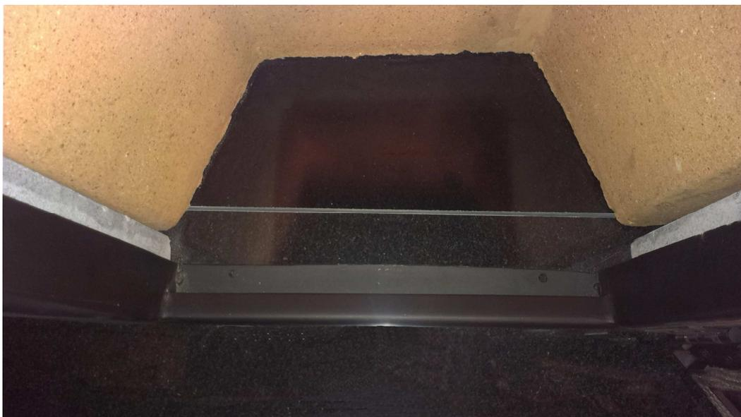
Use heat resistant sealant to fill the joint between the Fire Door base and the hearth.
