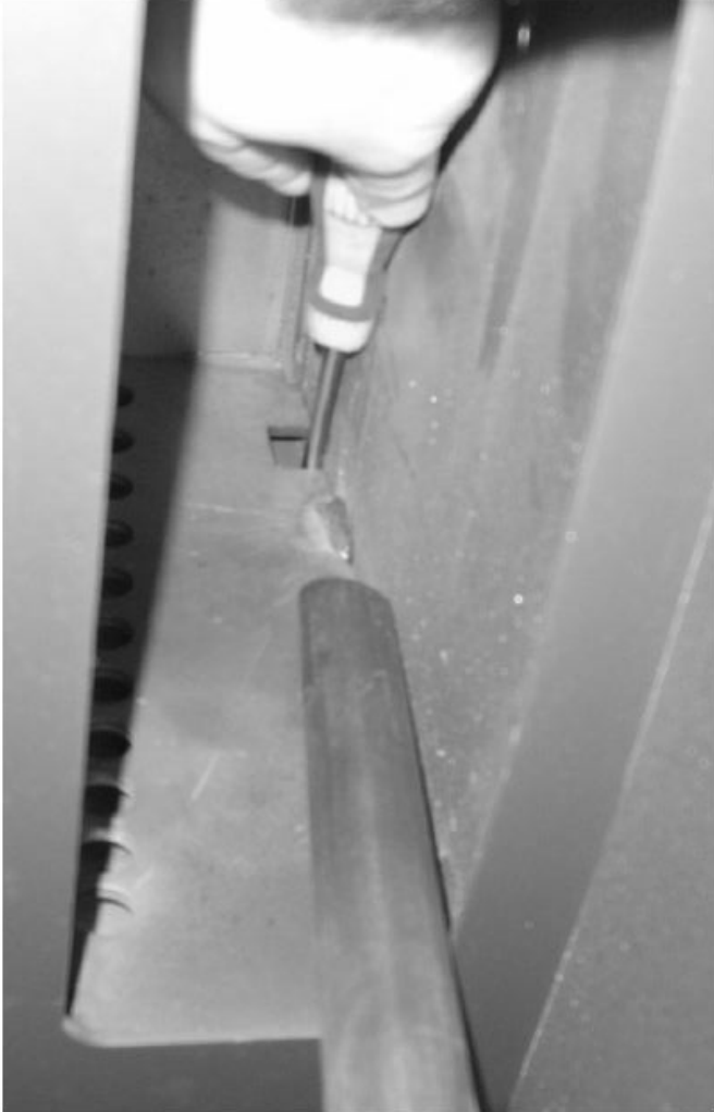
Figure 7: Removing ash from left hand landing cavity.
